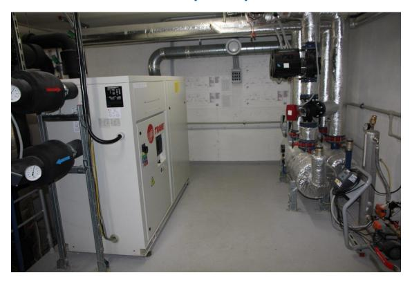
Heat pumps soil / water (Power 2 x 95 kW)
