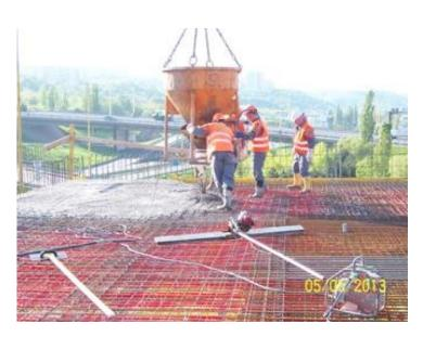
Heating and cooling by activation of the concrete core ceilings
