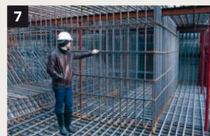
**5** Beams and stiffeners forming the grill, a view downstream
